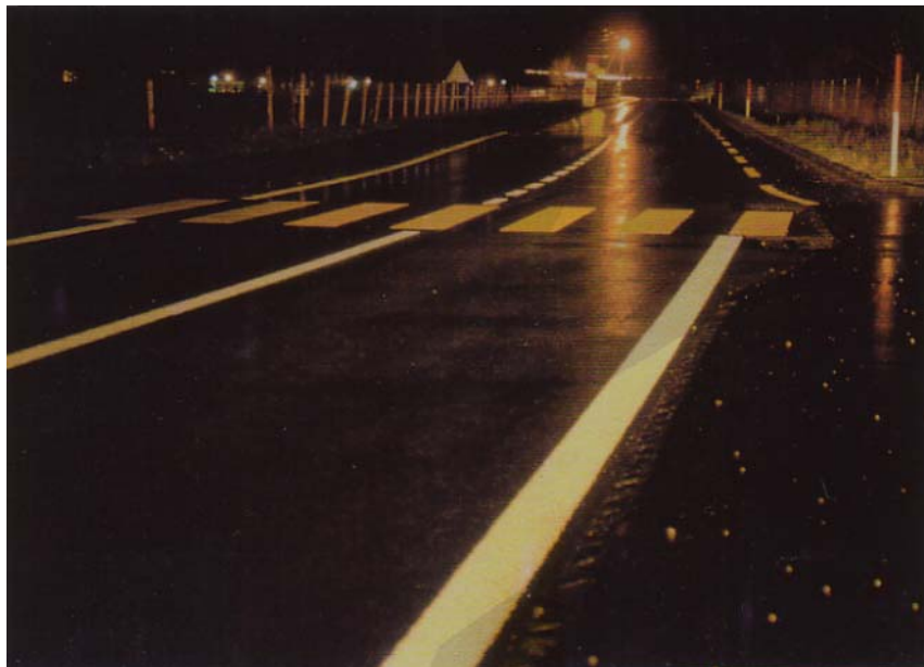
This picture shows an application-rate of 2 kg/m 2
