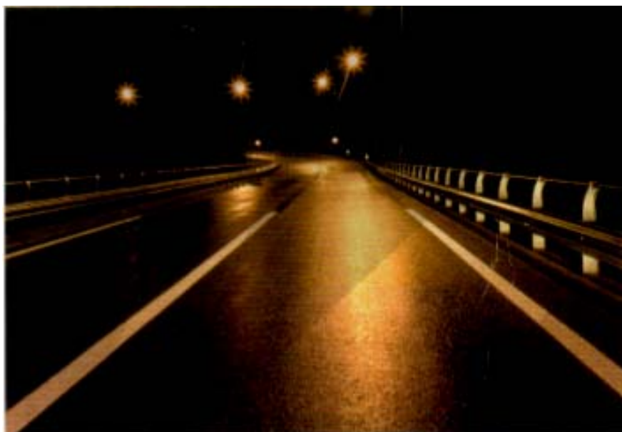
The Structure Road Marking stops in the middle of the picture at the State-border. The indistinguishable continuing lines are applied with paint.
